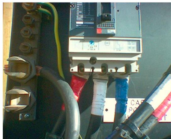
Incorrect method of termination, lugs have been modified - M12 (bolt/stud) not used
