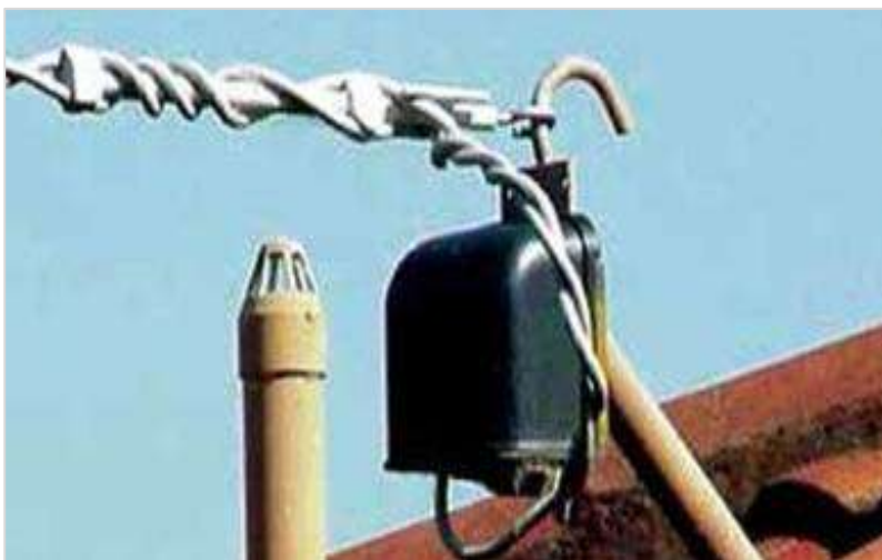
Figure 4.4 Sample image: twisted PVC service line
