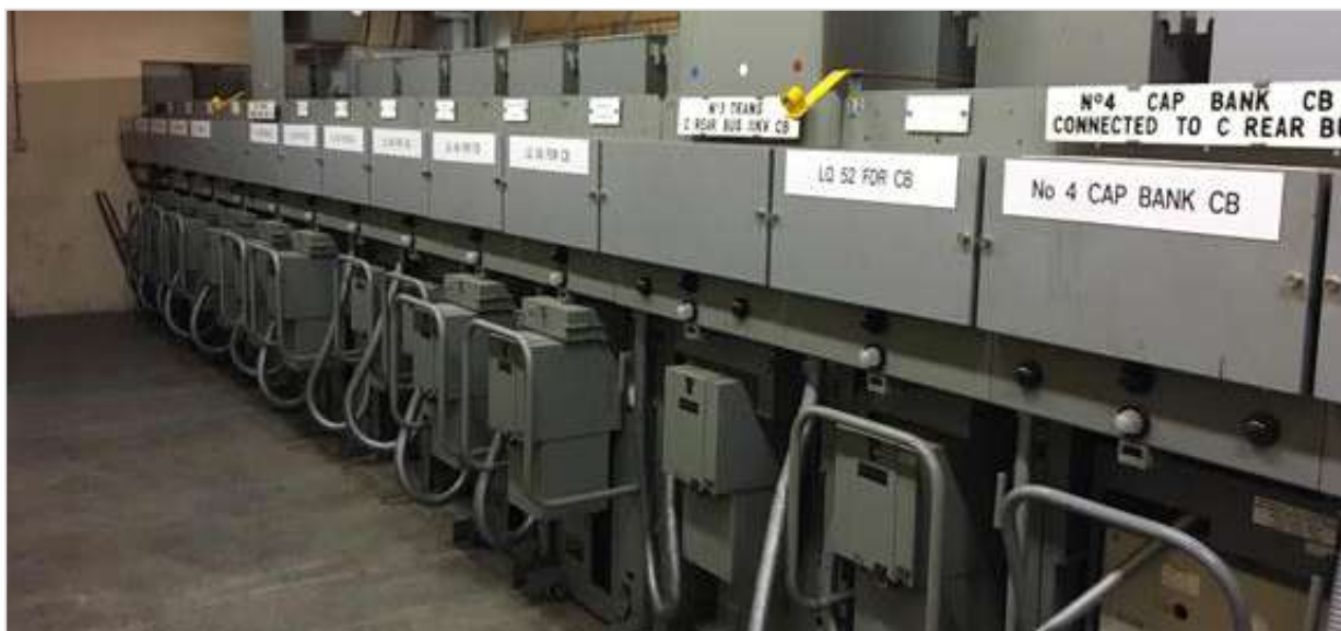
Figure 4.7 Little Queen zone substation: 11kV switchgear
