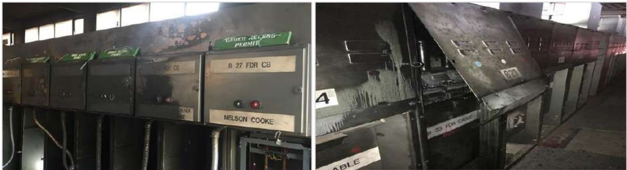
Figure 4.8 Damage to busbar chamber and switch room due to explosive failure at Collingwood zone substation (2016)
