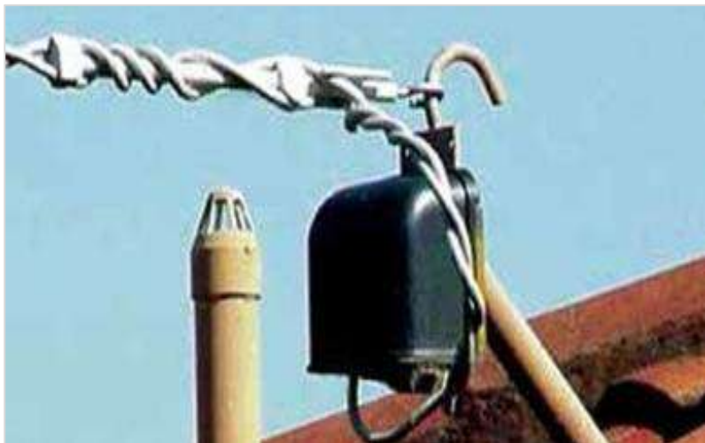
Figure 4.5 Sample image: twisted PVC service line
