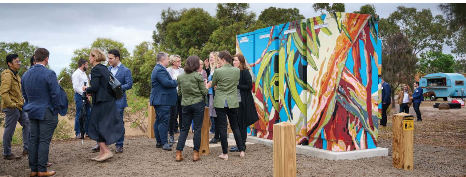
Powercor developed this 120kW (360kWh) battery in Tarneit to improve the network's capacity in a community with high rooftop solar penetration. This project was delivered with funding support from the Victorian Government's Neighbourhood Battery Initiative.
